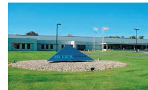
HI-LEX CONTROLS INC. LITCHFIELD PLANT (U.S.A.)
