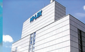
HI-LEX CONTROLS INC. LITCHFIELD PLANT (U.S.A.)
